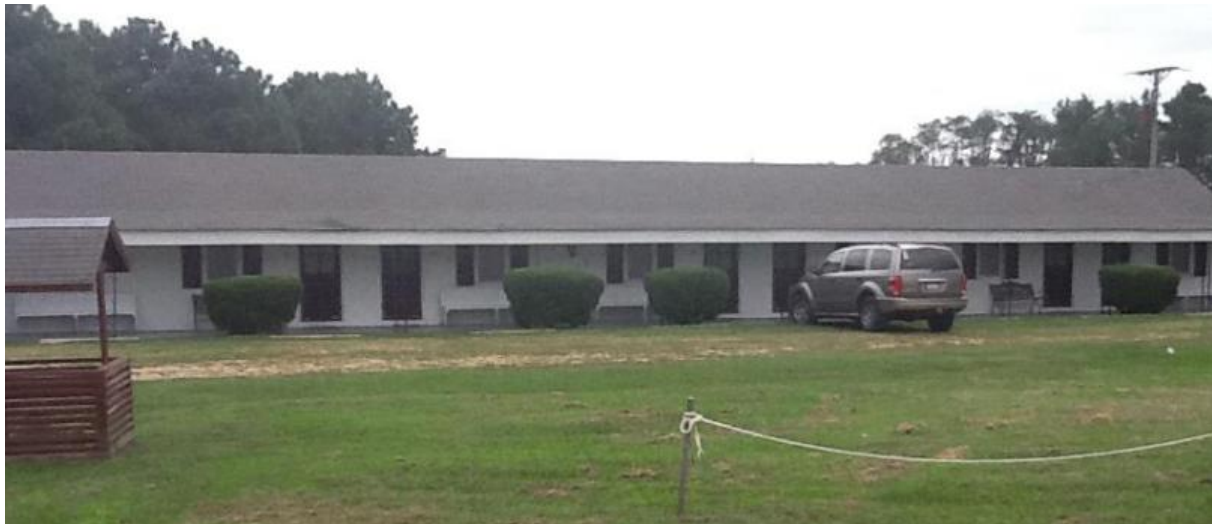
The motel rooms at Scheible's are undergoing a complete renovation.
