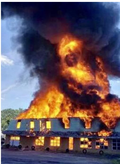
Fire destroyed a vacant commercial building in Leonardtown
