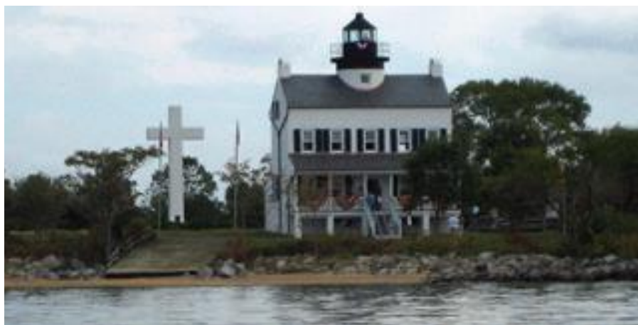
Blackistone Lighthouse will be closed this summer for repairs.
