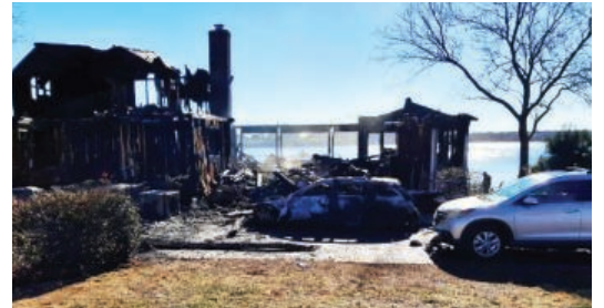
COPS & COURTS 13 Leonardtwn home destroyed by fire.
