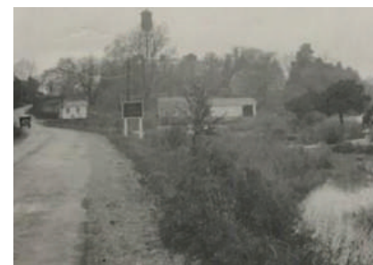
Route 5 at St Mary's City in the 1920s.
