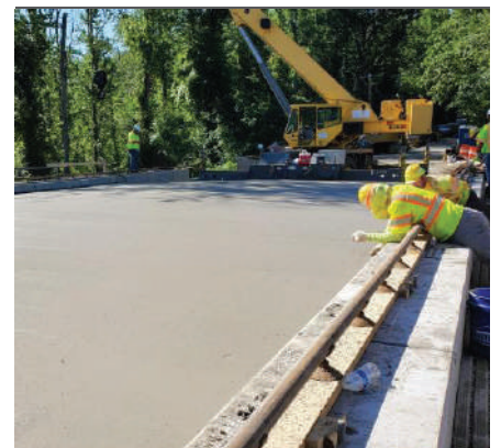
Concrete being laid at the MD 6 bridge over Persimmon Creek
