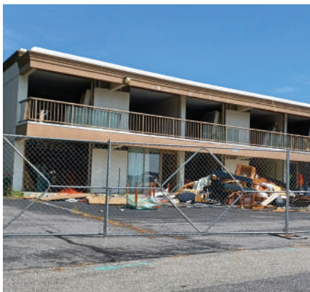
Demolition continues at the Pax River Hotel in Lexington Park
