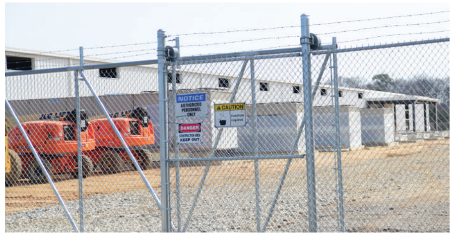
Medical cannabis growing facility currently under construction in Avenue
