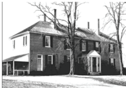
Tudor Hall prior to the 1969/70 renovations. Note 1st floor window to the right of the porch and absence of gutter and downspouts.
