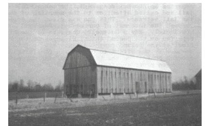
Gambrel Roofed barn
