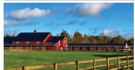
LOCAL 4 County seeks management help for Barns at New Market
