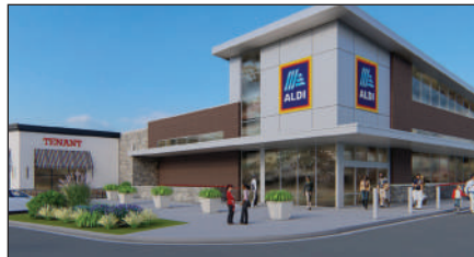
LOCAL 5 New grocery store signed for shopping center
