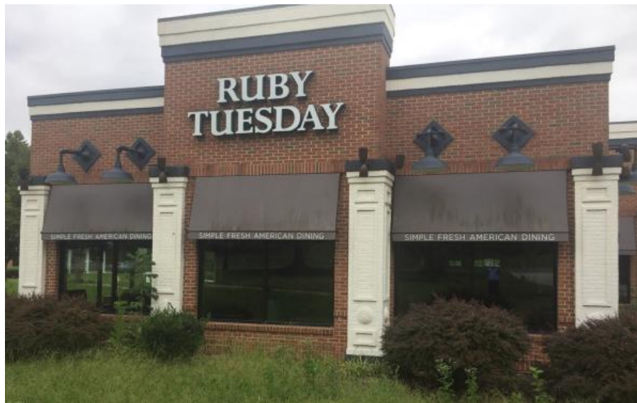
This closed Ruby Tuesday will be demolished.
