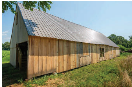
Recently stabilized Holly Hill Barn
