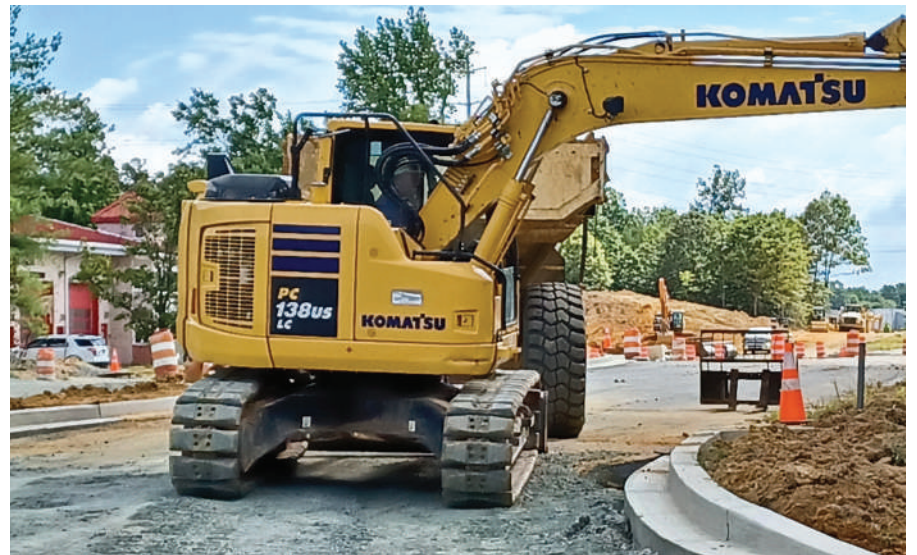
FDR Blvd at Chancellors Run Road and Fire Dept. Lane
