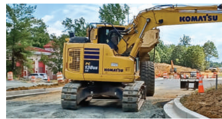
LOCAL 4 FDR Boulevard's next section under construction.
