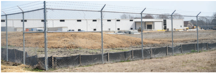
The Abell cannabis facility under construction in March
