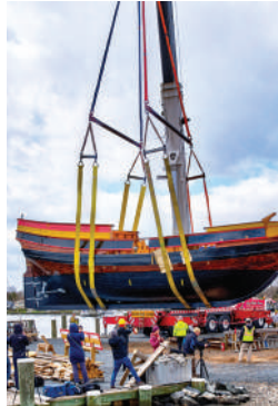
Construction of the new Maryland Dove
