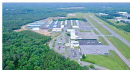
LOCAL 5 County shifts funding to airport improvements
