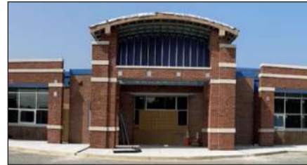
LOCAL 8 School renovations underway
