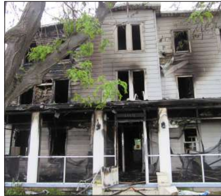
The charred remains of the Locust Inn after the April 2017 fire
